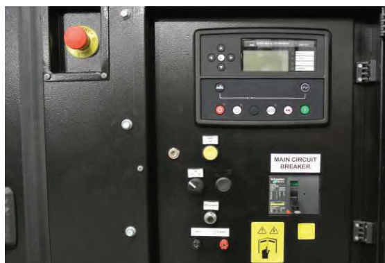
Control panel, with Deep Sea Controller, laid out and labeled for easy use. (other brands available)
