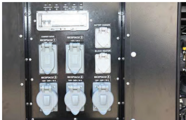
True 120V 20A outlet available in all phases.
