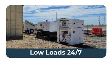
Reduce up to 80% of fuel burn and prevent generator damage that results from low load periods.
